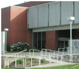
Ocean County College IT and Security Commissioning
