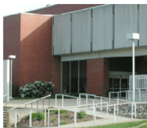
Ocean County College IT Commissioning
